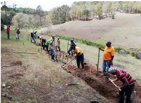
Infiltration ditches under construction by water users of the San Marcos de La Sierra community, El Platanar micro-watershed, Yamaranguila Intibucá (left). Irrigation groups and water board members of San Antonio Valle, Erandique building a series of stone walls to control erosion and sediment, La Chorrera micro-watershed (right).
